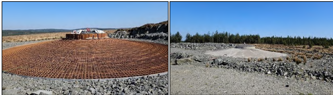
Plate 4-1 Turbine 'Anchor Cage' (left) and predominantly finished turbine base with only backfill outstanding (right)
