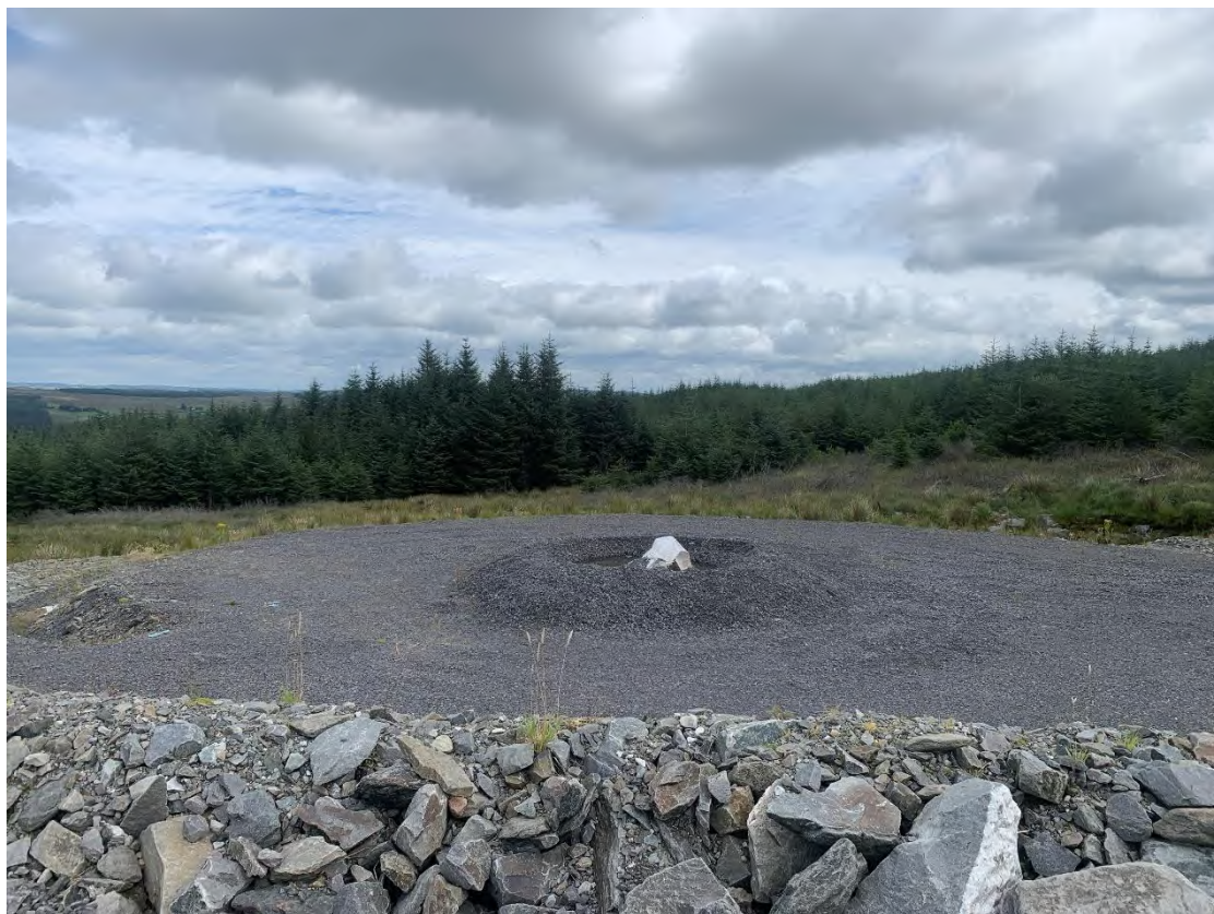
Plate 4-2 Finished Turbine Base located at T11, within the Wind Farm Site (bolts covered with gravel for protection)
